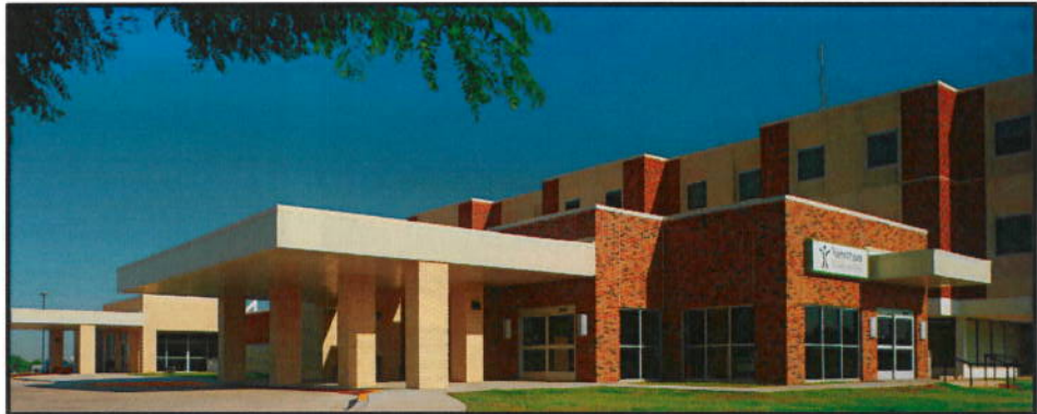
Newman Memorial Hospital 905 Main St, Ok 73858 580-938-2551
